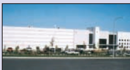
Zero Stantron's new facility in Valencia.
