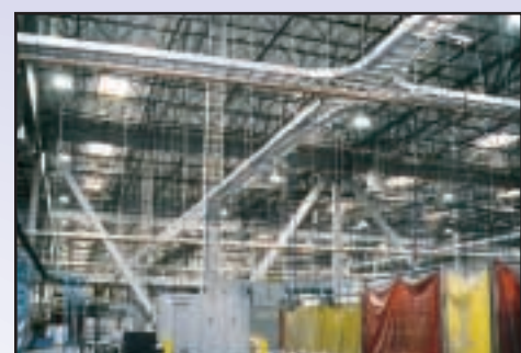
Cable tray installation.
