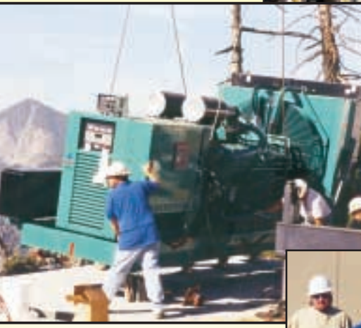
Lucian Tira's crew setting one of the 1250 KW generators.
