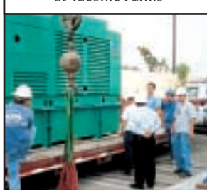
Installing a Diesel Generator at Taconic Farms
